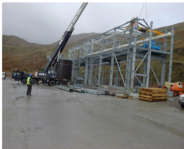
Installation of 2.1m 2 Filter Press—Foster Yeoman, UK
